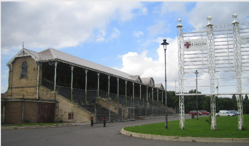
Fig. 16: The canopy roof of the Grade II listed grandstand at Lincoln Racecourse (1897) has charming daggerboard valancing
