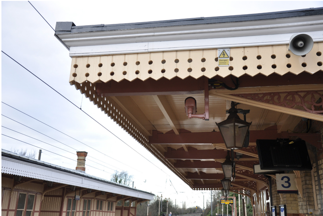
Fig. 10: Platform canopy fascias at the Grade II listed Hanwell Station, GWR 1877
