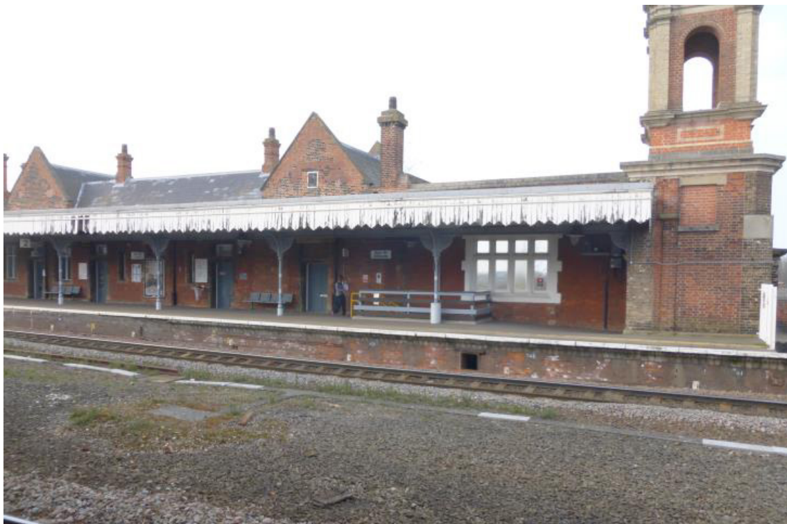
Fig. 6: The Grade II listed Bury St Edmunds station platform showing the timber platform canopy daggerboards in a poor state of repair before their replacement in FRP in 2016
