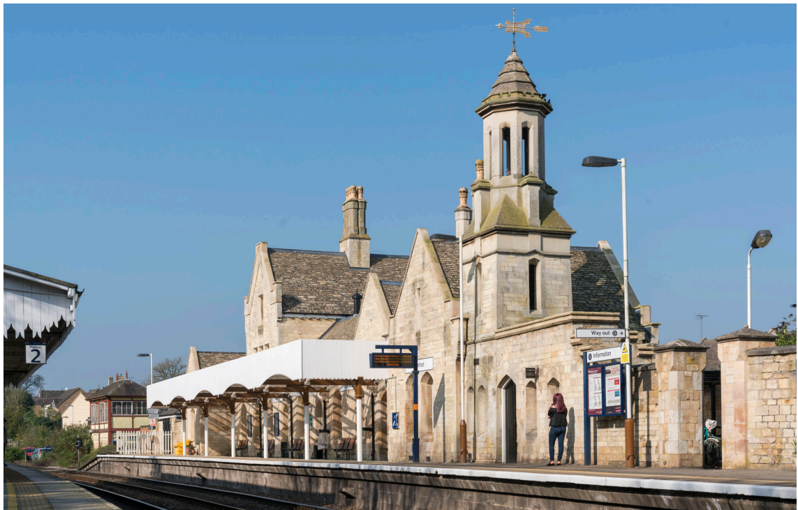
Fig. 12: The Grade II listed Stamford Station shown after the installation of FRP canopy valancing in 2017
