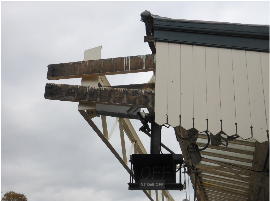
Fig. 7: Newport Station platform canopy pictured in 2016. The canopies required cutting back due to the electrification of sections of the Great Western mainline route
