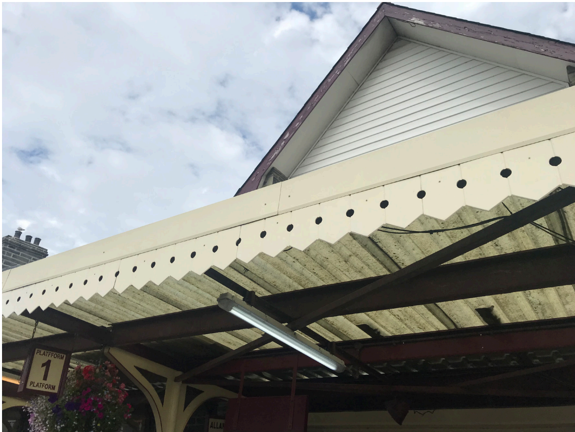
Fig. 9: FRP valancing was used on the canopy at Porthmadog Harbour, on the Ffestiniog Railway, more than thirty years ago. Though this level of installation is not acceptable today, it serves as an example of the structural and aesthetic durability of FRP in an aggressive seaside environment
