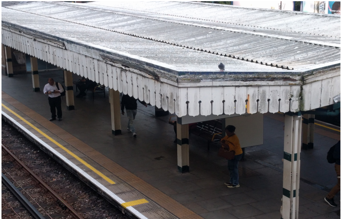
Fig. 1: Timber station canopy valancing at Finchley Central Underground Station (1867), pictured in 2016
