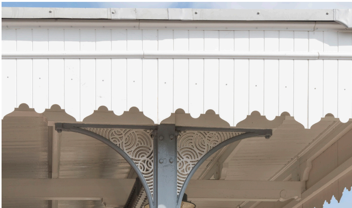
Fig. 8: FRP fascia daggerboards at the Grade II listed Bury St Edmunds Station
