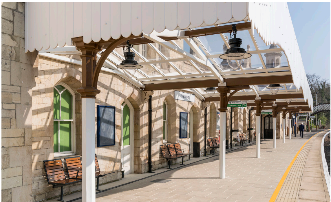
Fig. 13: A closer view of Stamford Station's FRP canopy valancing
