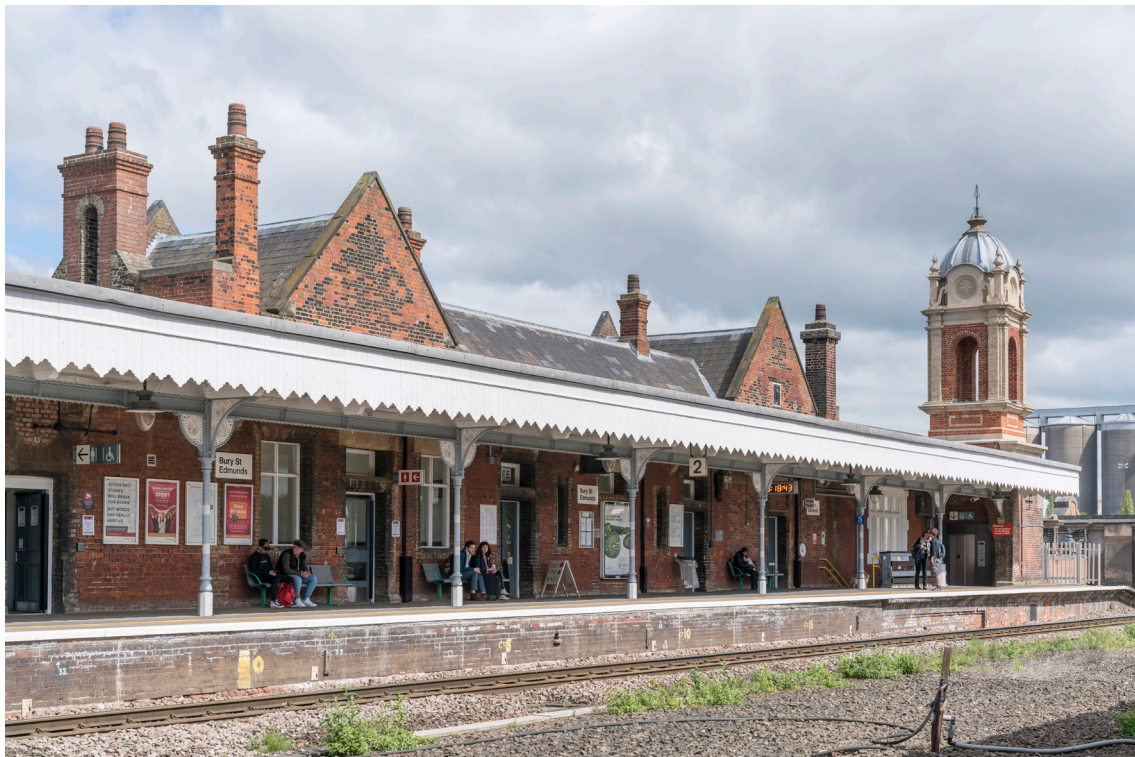
Fig. 11: Bury St Edmunds station platform pictured in 2018 after the timber canopy daggerboards (Fig 4) were replaced with FRP
