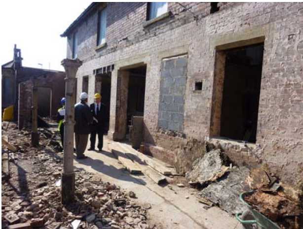
Work in progress at Moorthorpe
