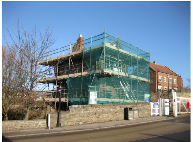
Work in progress at Bedale
